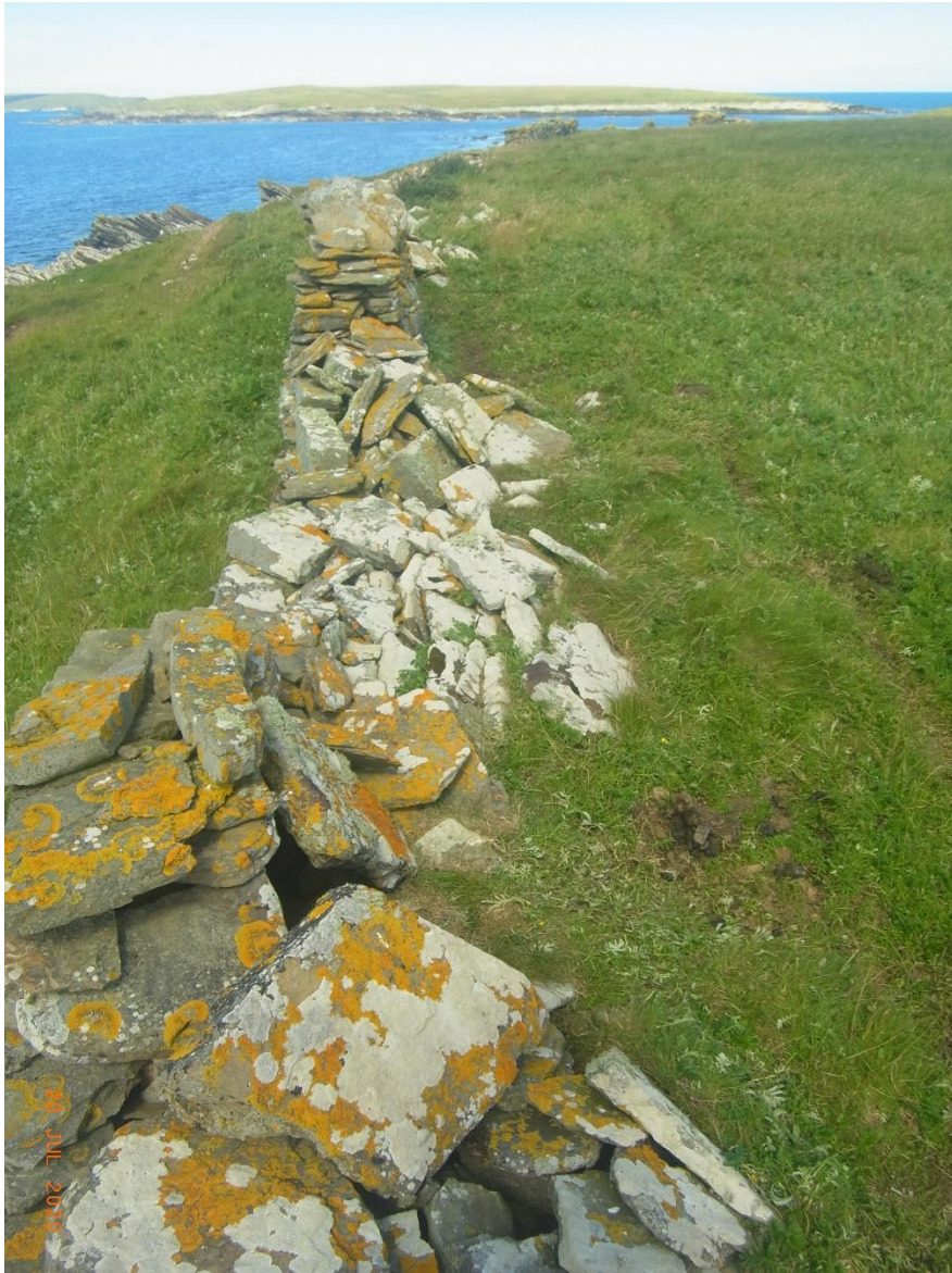
Calibration zone from West – Stone Dyke
