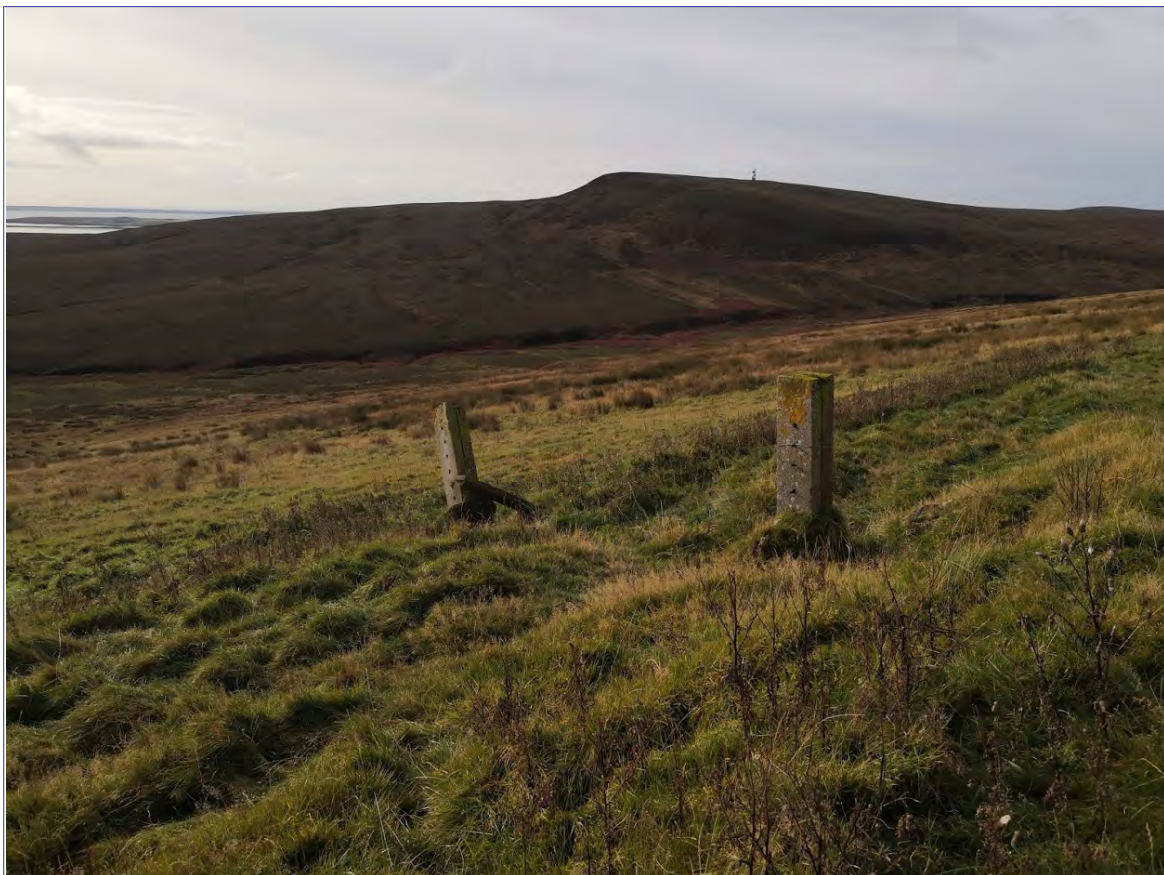
Plate 8: Concrete gate piers (Site 495) marking southern edge of Second World War military site
