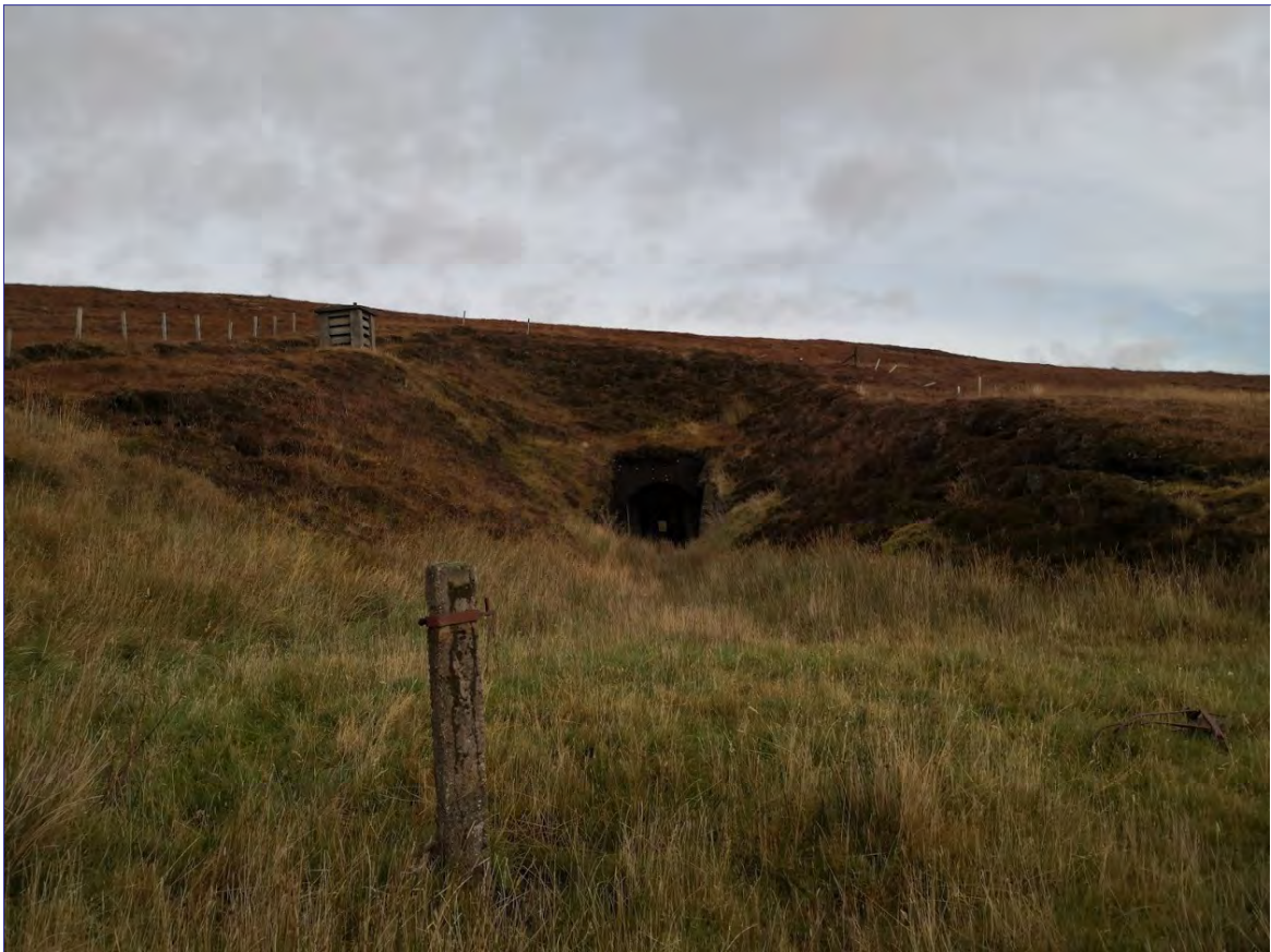
Plate 16: Secondary entrance to Underground Fuel Reservoir (Site 143) from north-east
