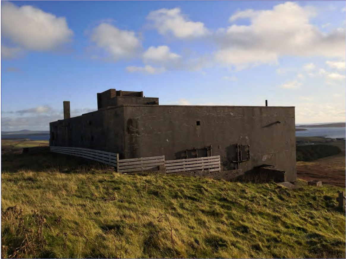
Plate 13: Category A Listed Former Naval Command and Communications Centre (Site 127) from south-west
