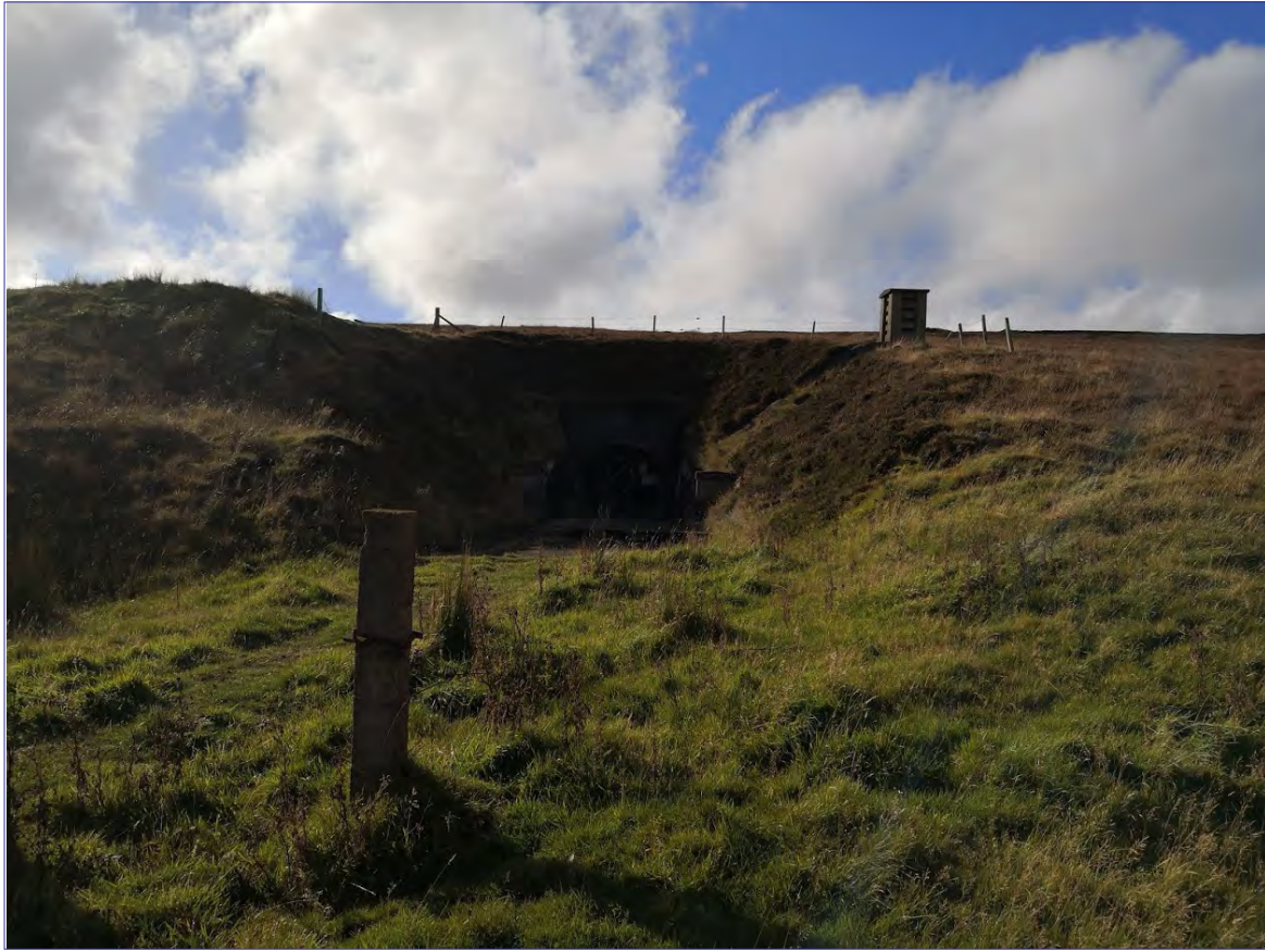
Plate 17: Principal entrance to Underground Fuel Reservoir (Site 143) from south-west
