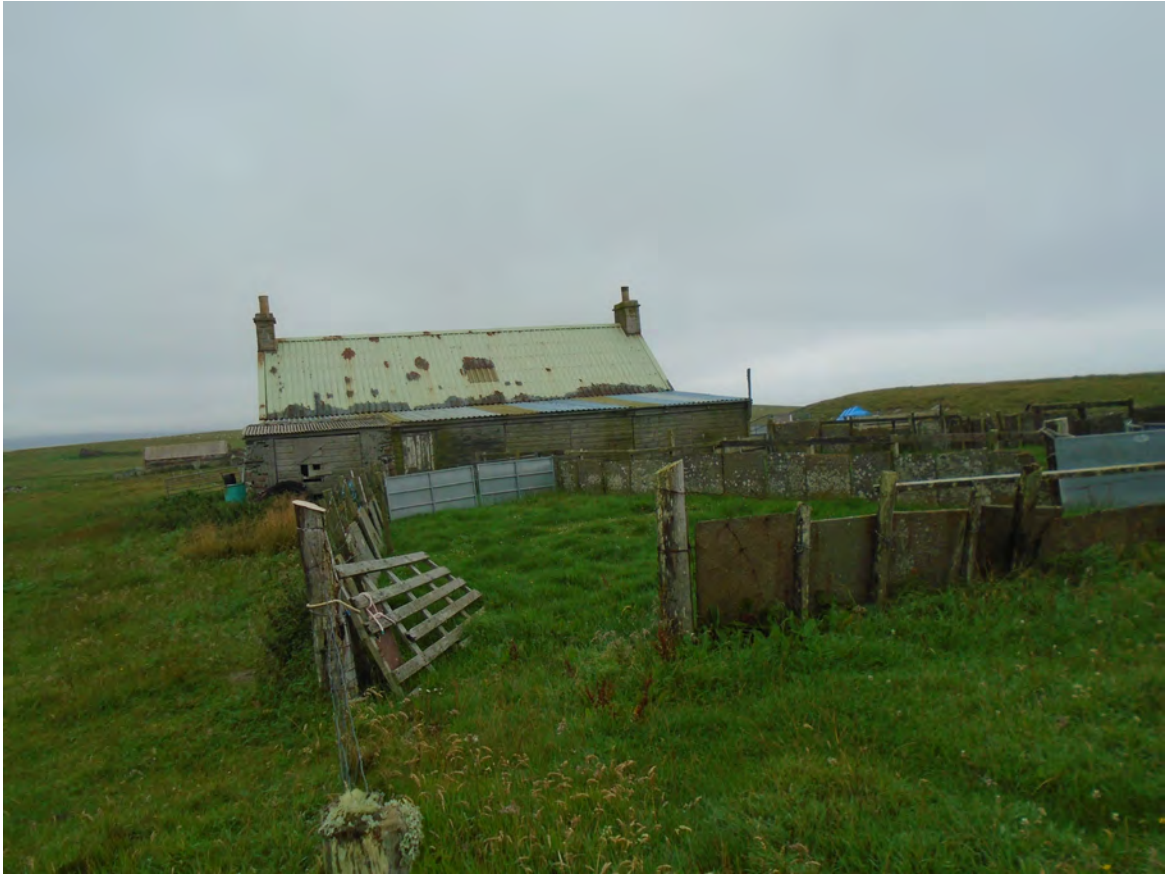
Plate 21 Rear of school (Site 54) and flagstone fence from north
