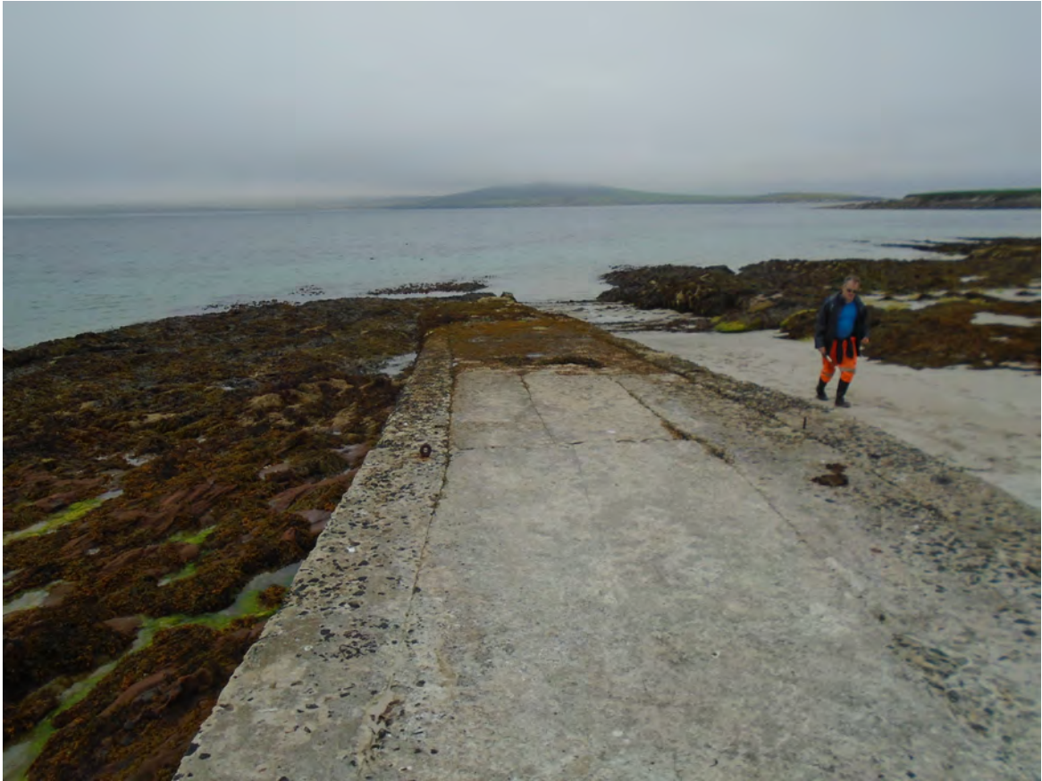
Plate 33 Concrete slipway (Site 119) from north-west
